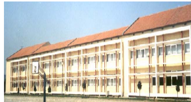
Figure 19. High School (Valongo do Vouga)
